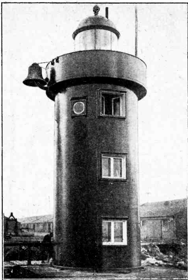
The lighthouse from which the bell is sounded, showing the lens window which receives and concentrates the beam.
