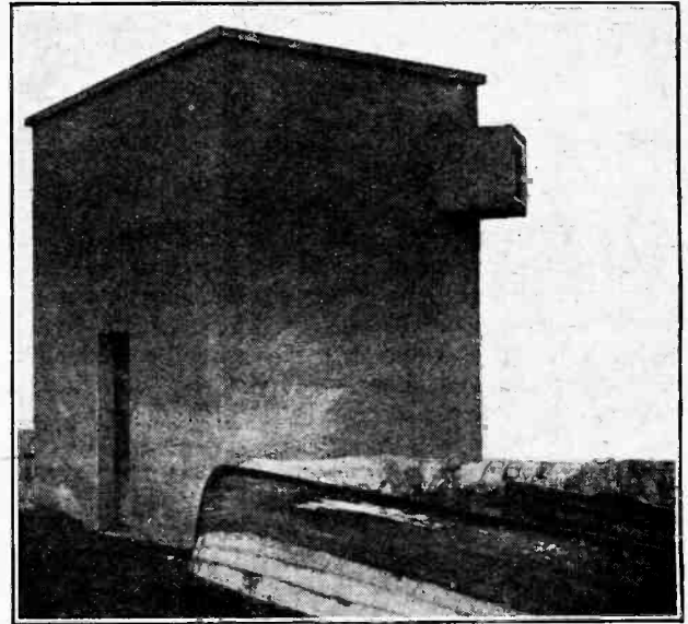
The lamp house. The light emerges from the square window on the right. Actually two lights have been installed in this building working with two independent light-detecting equipments.
