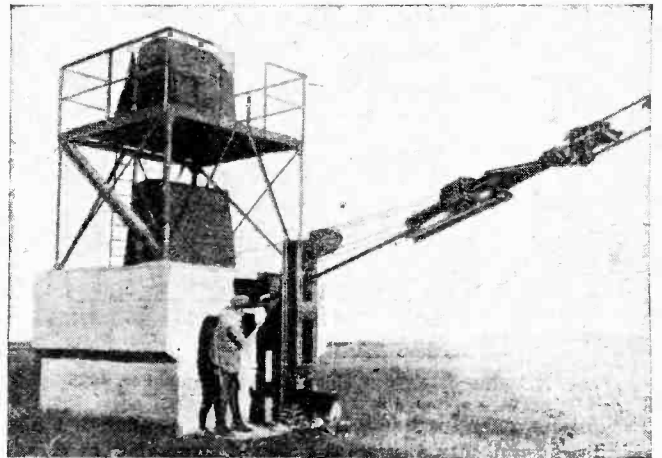
One of the massive stay wire anchorages.
